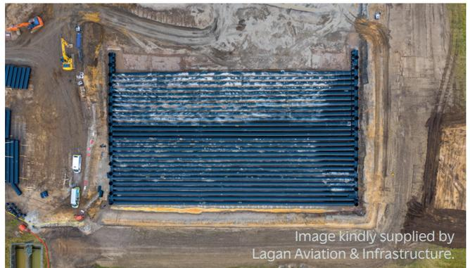
**Malachey Doyle, Project Manager, Lagan Aviation & Infrastructure, said:** *“Safe, tidy and impressive work rate by all within our Central and Eastern section at RAF Lossiemouth. Works have comprised a new wastewater treatment works, 90m x 90m oversized attenuation tank, roads, drainage and associated Infrastructure.”*
